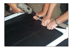
7 Place one screw in the mid point of the PVC and screw the cloth to the PVC.
